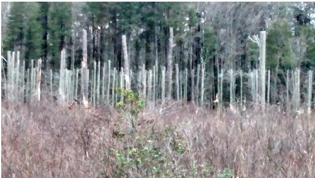
Figure 9: Trees topped in a span. The prescription for this wetland span requires hand cut and removal of trees by hand in late summer. However, concerns over wetlands impacts caused by vehicles needed to remove the trees from the span and impacts to the newly Federally listed Northern long-eared bat lead a utility company to request a prescription timing window modification and to perform tree topping instead of the ROW Plan prescription.
